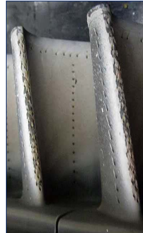
(b) Erosion of leading edge.
